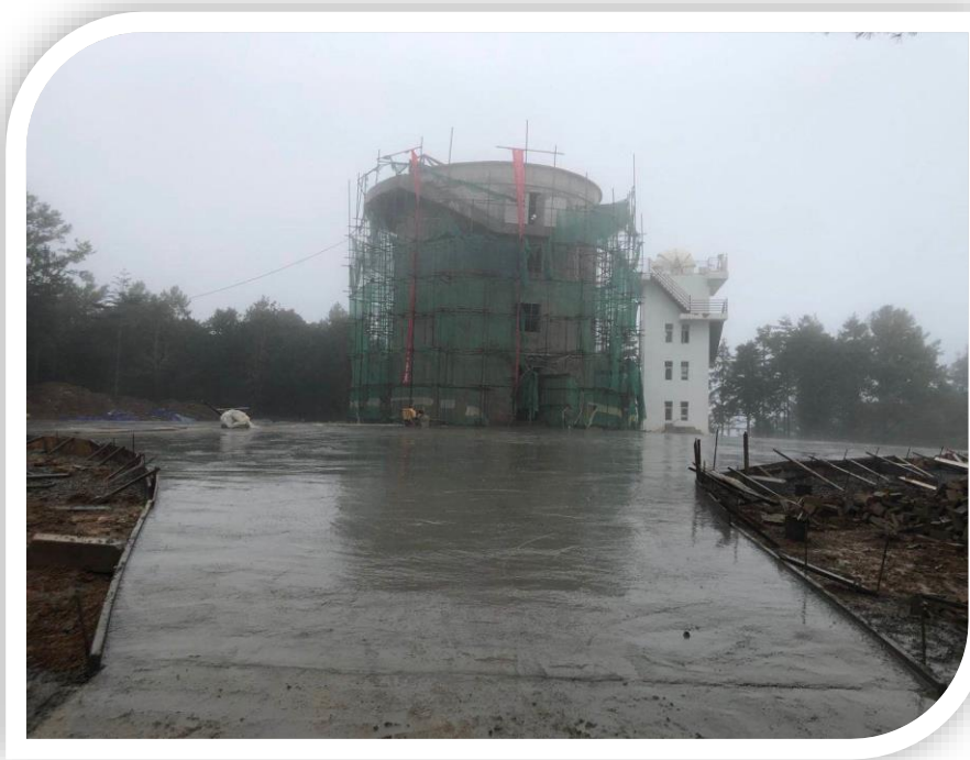
图 3.9：目前主体工程外观图 Exterior view of the telescope main building
